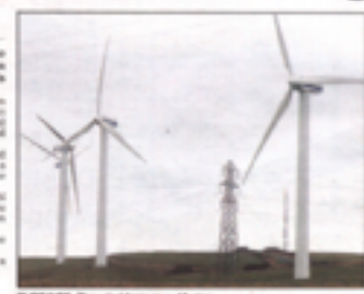
TURBINES: The wind farm near Morton
