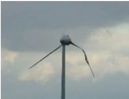
Louth, Lincolnshire, January 4th, 2009. The blades hit the Ecotricity Enercon turbine tower and one was thrown clear.
